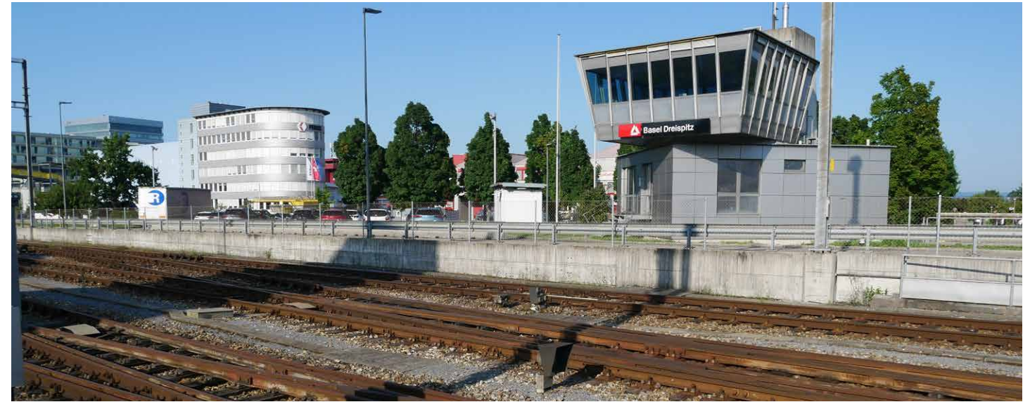
Former signal box Basel Dreispitz
